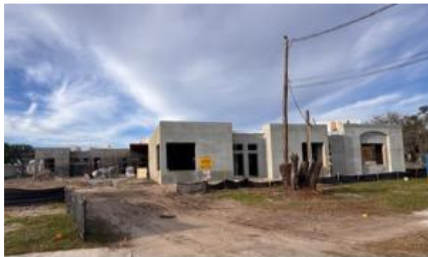
(Construction progress of the early childhood center as of March 2026.)
